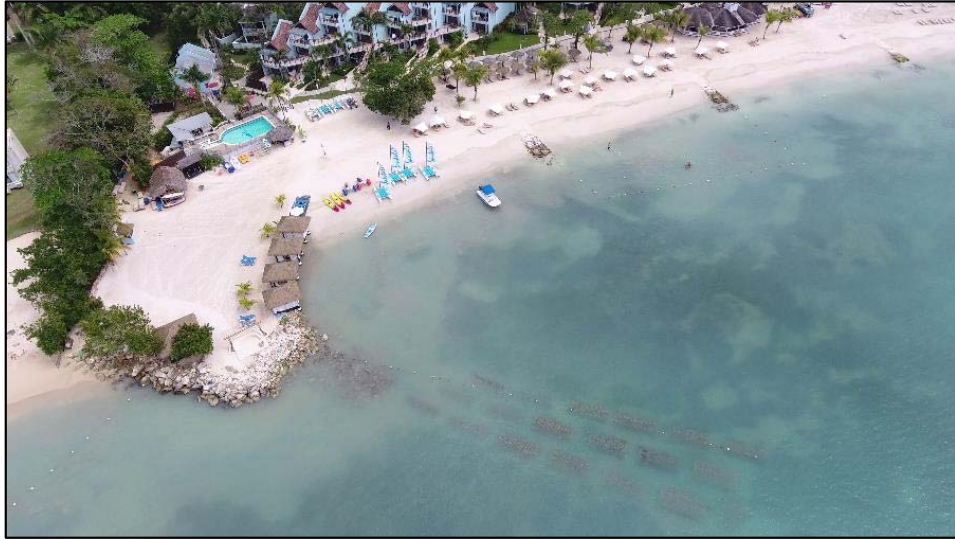
FEB 2022 16 Months Post-Construction
